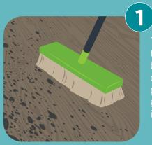
Thoroughly clean the subfloor with a broom or a vacuum cleaner, removing paint residuals or glue from earlier installations
